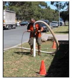
**P.D. Excavations** provides *underground service locations* and *vacuum excavation* in South Australia.
