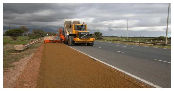
**P.D. Excavations** is equipped with two road wideners, capable of placing material on road shoulders up to 3 metres wide. Automated machine controls are fitted to ensure precise placement of material to exact customer specifications.
